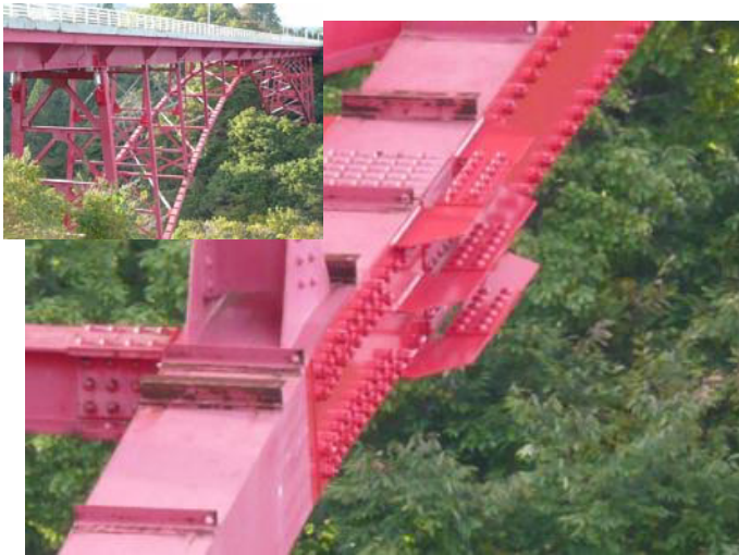
Photograph 13. Strengthening a steel truss bridge
