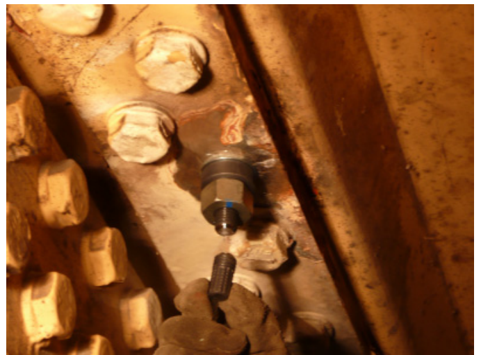
Photograph 16. Replacement of OS-Bolt
