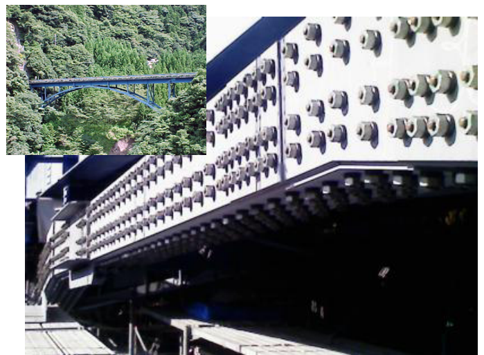
Photograph 11. Strengthening a steel arch bridge
