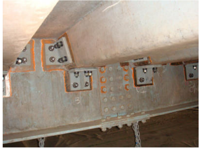
Photograph 15. Strengthening a U-Rib of steel slab
