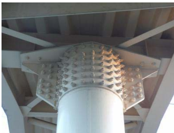
Photograph 5 Strengthening a steel pipe piar
