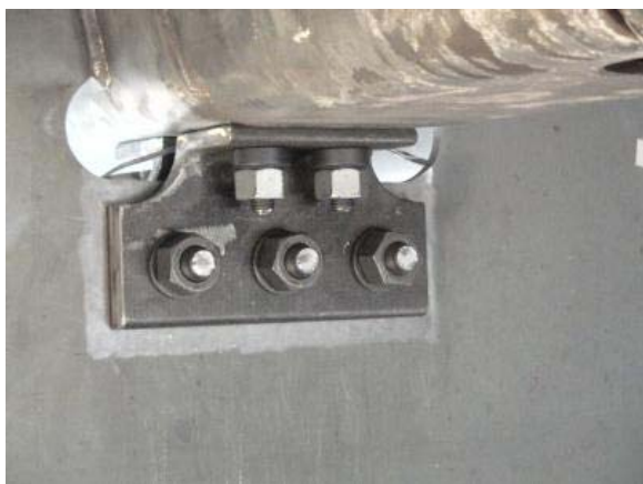
Photograph 4 Strengthening a steel slab U rib
