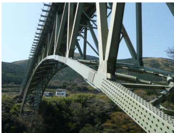
Photograph 3 Strengthening a steel arch bridge
